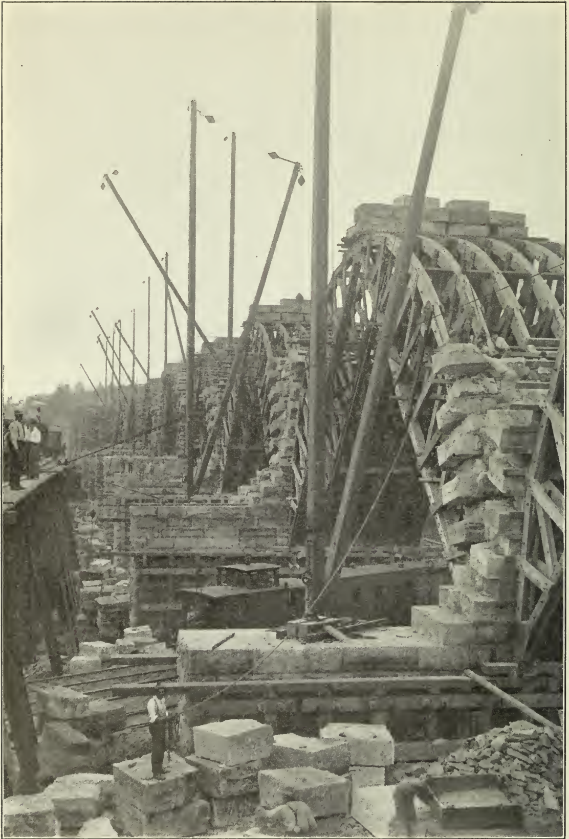
BUILDING THE NEW BRIDGE AT COATESVILLE, PA.
